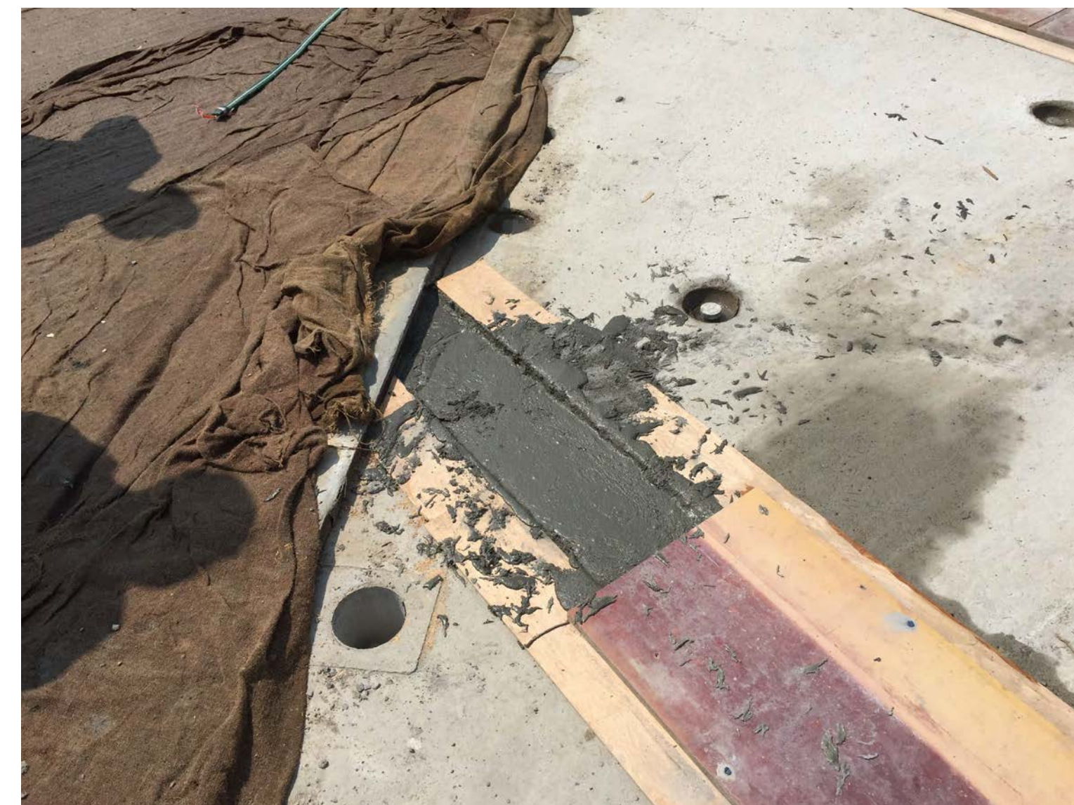
Concrete for over-pour and formwork
