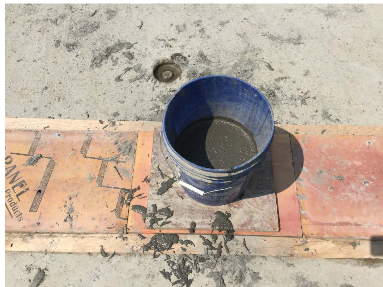
Concrete for over-pour and formwork
