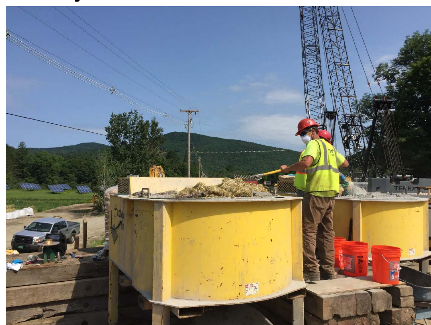
Shear mixer and bags of cement mix to be combined with water
